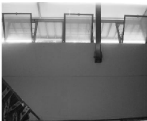
Fig. 1. Windows of hospital ward flipping inward
